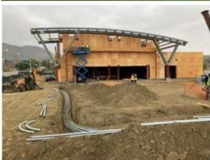
Fuel Station electrical trenching and installation.
