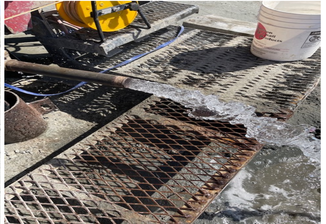
Testing the water @ 20 GPM
